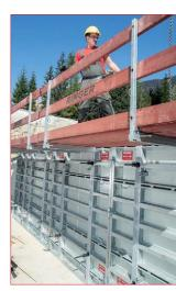
Concreting platform "L" Lenght 2.70m
