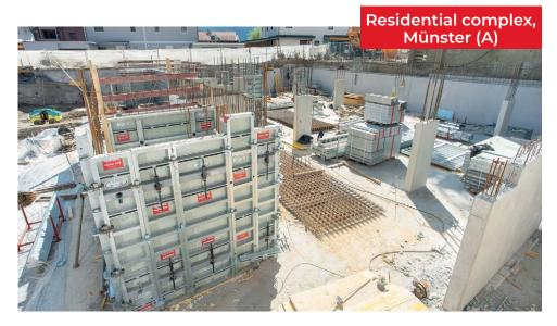
Thanks to the tie rod storage space, the tie rods are always where they should be.
