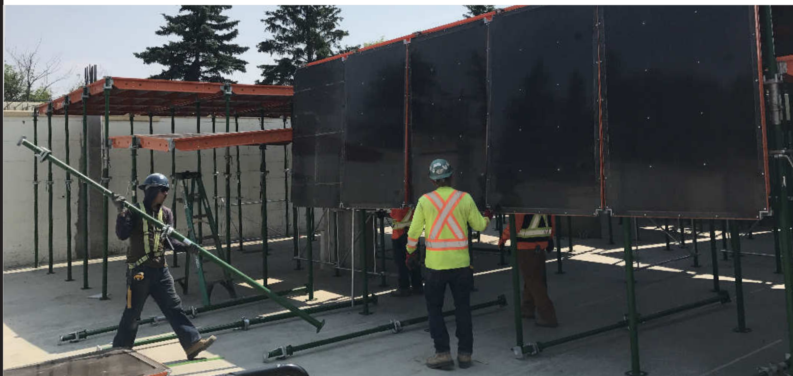
Swing the lower end of the panel into position.
