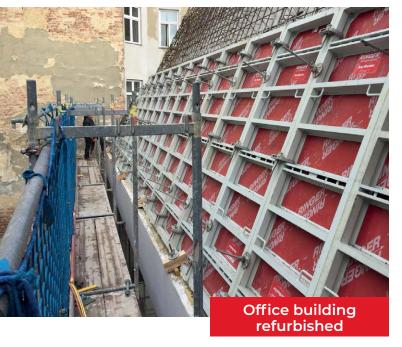
Alu Master equipped with plastic plywood- also suitable for inclined applications
