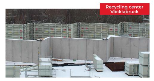
The retaining wall was formed using Alu Master panels with Alkus plywood
