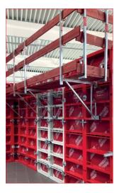
**Concreting bracket** with railing
