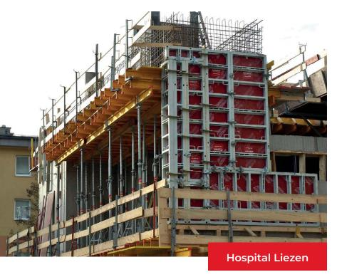
Alu Master panels can be combined as desired, which makes them readily adaptable to any layout.
