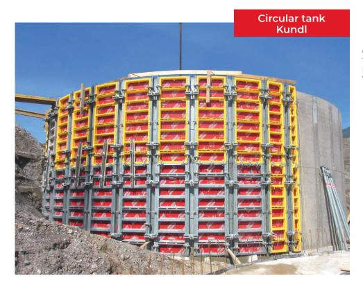
In combination with the Master circular forming plate, round tanks are quickly formed. In the picture Alu Master is combined with Steel Master.
